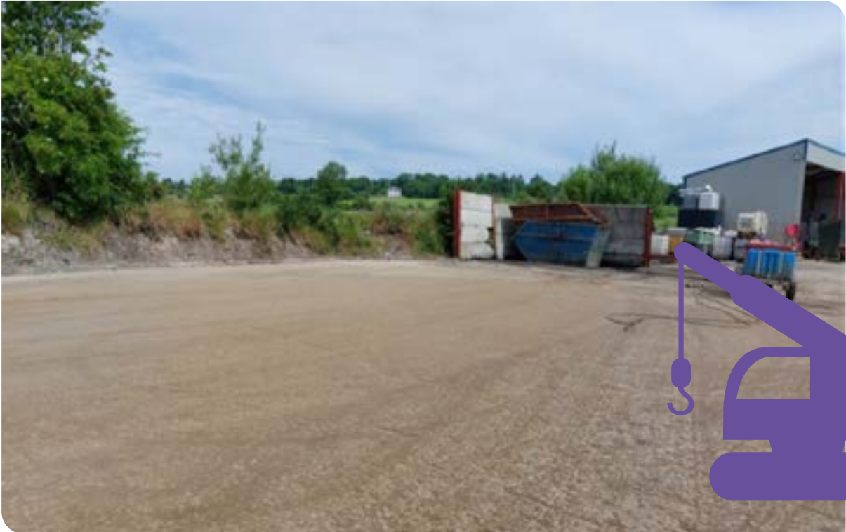
Photograph 3: Site restored and clean
